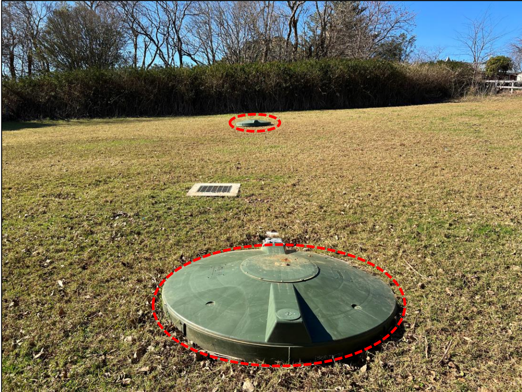
Site Photograph 6.7.3 Underground septic tanks, located within paddocks north of residential structures, viewed facing east.
