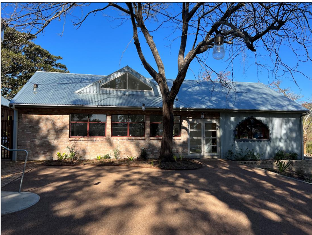
Site Photograph 6.2.4 Sheet metal and brick venue hall, located on the southern boundary of the site, viewed facing south.
